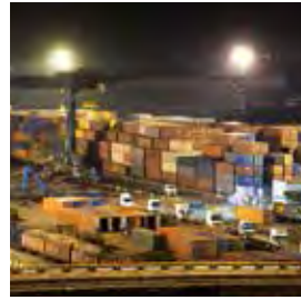
7 Area Lighting/ Truck Parking Area
